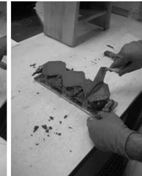
6. Cut off Mortar By Drawing Trowel with A Sawing Motion.
